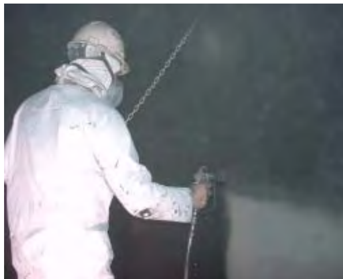
Spray application of FlueGard™-425S
