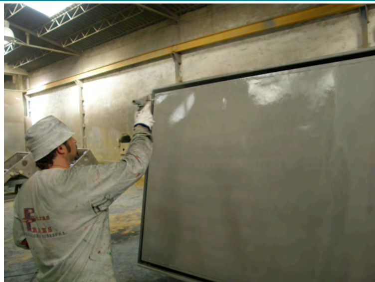
Spray application of CorrosionGard™-160S
